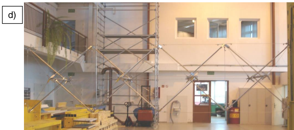
Fig. 4 a) Single octahedral module in a graphical form (a three-dimensional shape with eight equal triangular faces), b) Structural solution of the active cable with nodes located inside each of four tensegrity modules, c) and d) Class \Theta tensegrity girder as a deployable and modular tensegrity column or beam depending on actual needs.
