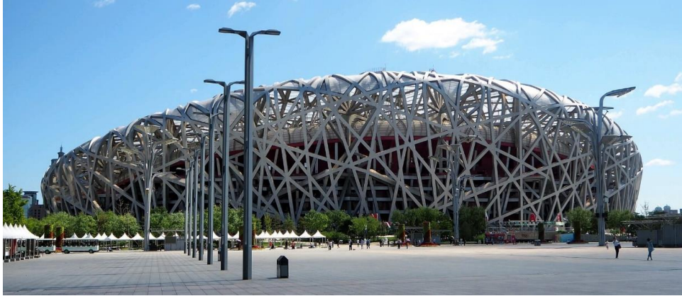
Fig. 2. Beijing National Stadium 'Bird Nest' 2003 – 2008. Artistically inspired by crackle-glazed Beijing pottery and heavily veined Chinese scholar stones. Deconstructivism style; cost: $345 M - $423 M; 420,000t of steel and 110,000t of concrete used, giving an estimated total of CO 2 : 800,000t (5 times that of the Wembley Stadium, London, of similar capacity)
