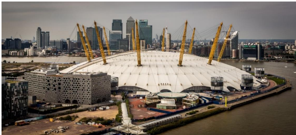
Fig. 3. London Millennium Dome 2000. Teflon-coated glass-fibre membrane on pre-stressed cables supported by masts via stay cables; an unnatural choice of form for a surface-stressed structure, huge forces present at the top of the membrane, stay cables proved too short to mate with the surface during construction (as the membrane crept towards its minimal form), saddling of the surface not eliminated
