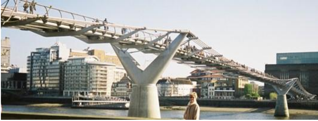
Fig. 4. London Millennium Bridge 2000. Architecture: Norman Foster, Engineering: Buro Happold; light aluminium deck prone to lateral vibrations. nearly horizontal suspension cables generated extremely high tension forces (22500kN) as in a suspension road bridge, equal length cables acted as guitar strings encouraging vibration, structure retro-fitted with dampers (at an additional cost of £5 M) to eliminate lateral sway
