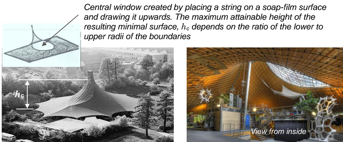
Fig. 6. IL Tent, Stuttgart 1965; a listed building. Design: Frei Otto/ Atelier Warmbronn utilised cable net and soap-film models
