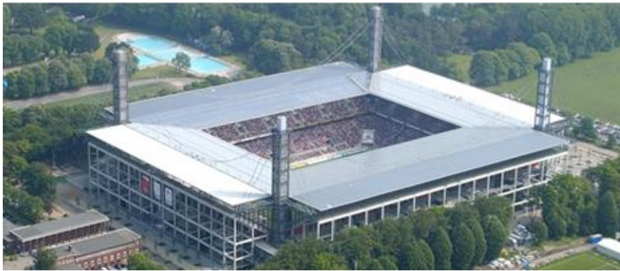
Fig. 13. Complete roof of Cologne Stadium.
