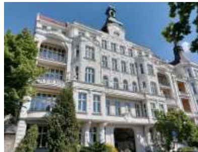
The facade of the building of the Wrocław Branch of the Polish Academy of Sciences
