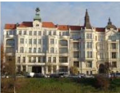
Building of the Wrocław Branch of the Polish Academy of Sciences
